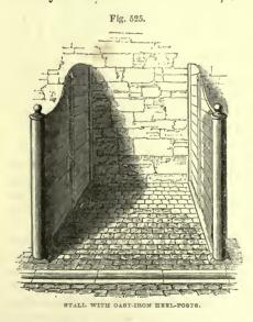
1288. Fig. 525 is a specimen of a stall for a work-horse stable, with cast-iron heel-posts.
