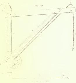
be  $\frac{1}{2}$  inch diameter, which is sufficient, if of proper quality, to bear a load of 2 tons; it passes from the barrel upwards, and over a pulley k; supported on brackets at the point of the jib, and is provided with a strong hook l at the end, for attaching the load.
