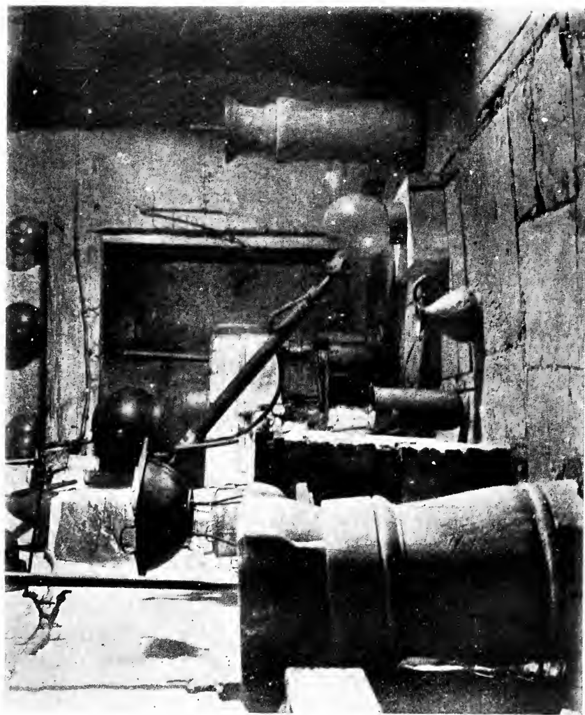
OLD LABORATORY AT MR. HOOPER'S, 24 RUSSELL STREET, COVENT GARDEN. THE LARGE STILL IN THE CORNER IS FOR DISTILLING ROSE AND AROMATIC WATERS THE SMALLER STILL IS FOR DISTILLING SPIRIT ESSENCES
