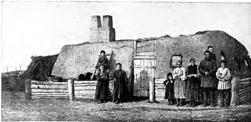
A YAKUT WINTER HOUSE, WITH SLOPING TIMBER WALLS AND ROOF OF CLAY AND PEAT
