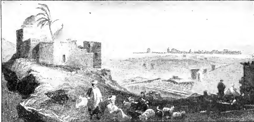
FROM THE MAINLAND SHOWING RUINS OF AQUEDUCT TO THE ISLAND
