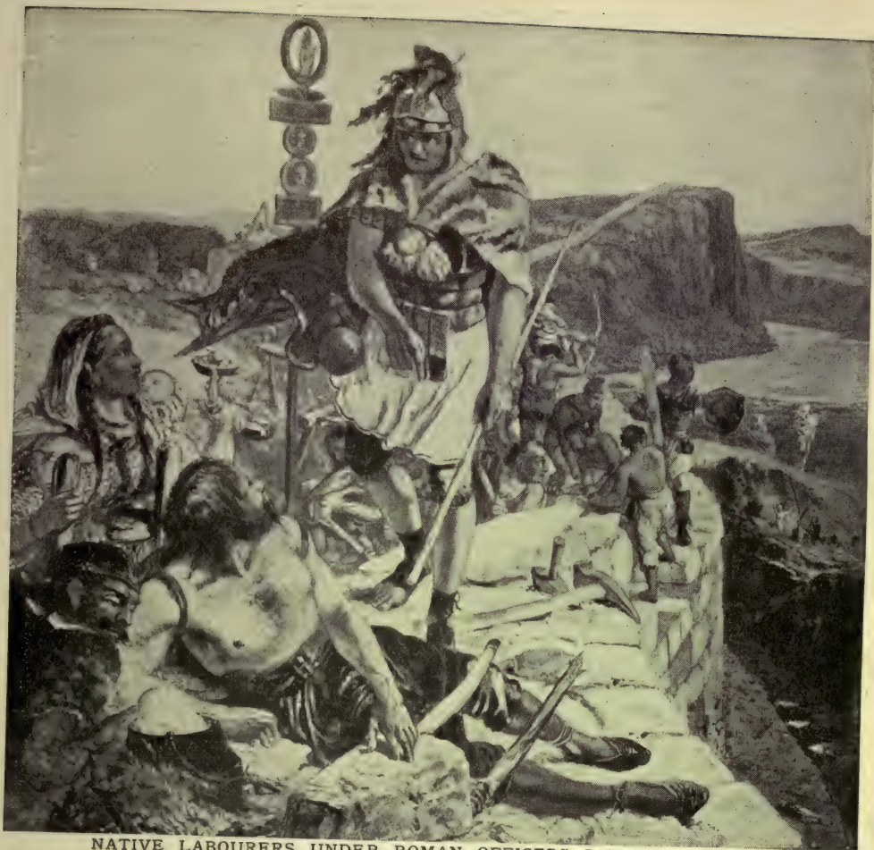
NATIVE LABOURERS UNDER ROMAN OFFICERS BUILDING A WALL From the fresco painting by William Bell Scott
