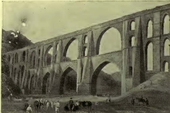
AQUEDUCT OF THE GREEK EMPERORS, NEAR PYRGO
