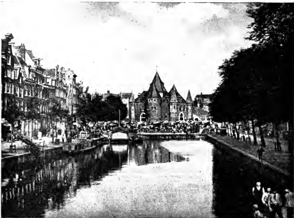
THE NEW MARKET AND OLD WEIGH-HOUSE, BUILT AS A TOWN GATE ABOUT 1488
