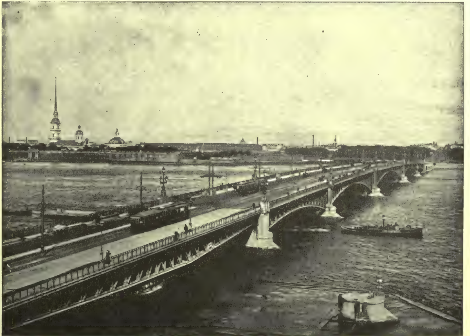
THE OLD ADMIRALTY BUILDING FROM ONE OF THE BRIDGES SPANNING THE NEVA PETROGRAD, THE MODERN CAPITAL OF THE RUSSIAN EMPIRE
