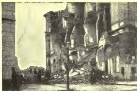
THE DAMAGED POST-OFFICE
