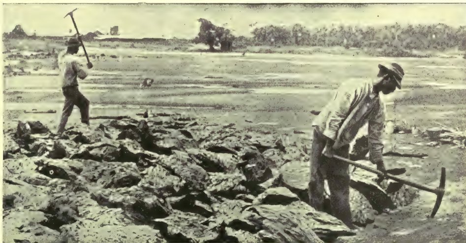
NATIVES DIGGING THE PITCH
