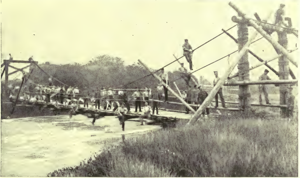
MEN OF THE ROYAL ENGINEERS CONSTRUCTING A SUSPENSION BRIDGE
