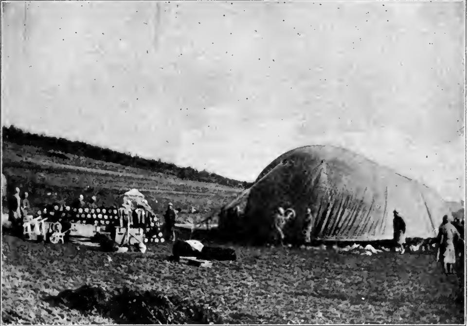
INFLATING A BALLOON FROM CYLINDERS OF HYDROGEN GAS
