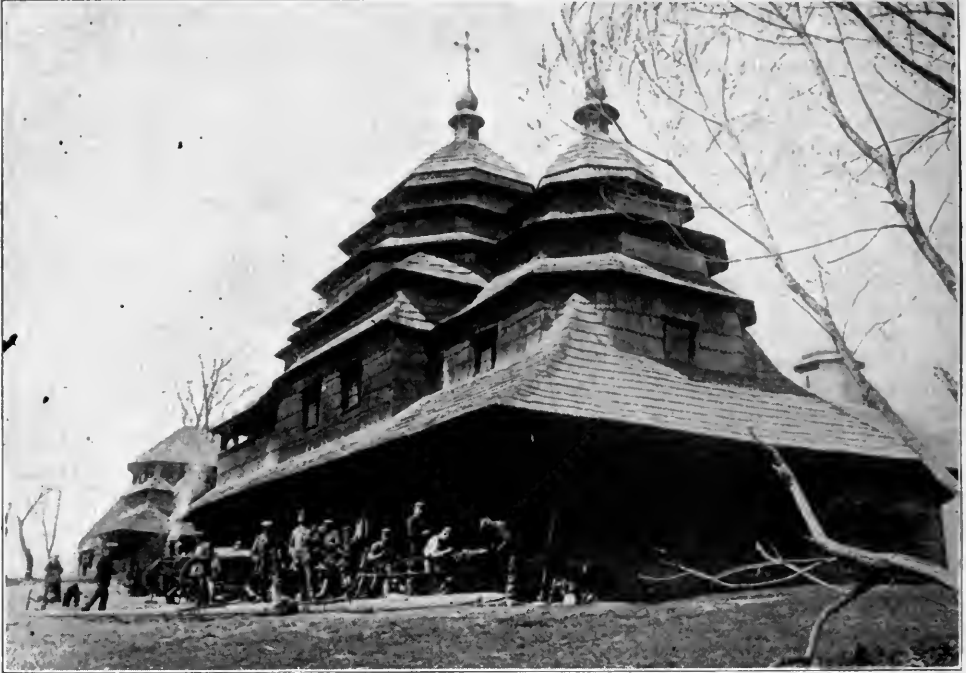
A TYPICAL RUTHENIAN CHURCH TRANSFORMED INTO A WORKSHOP
