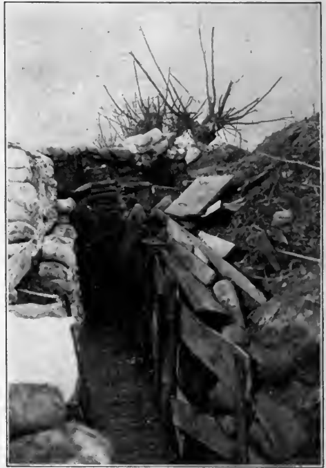
A TRENCH NEAR ARRAS
