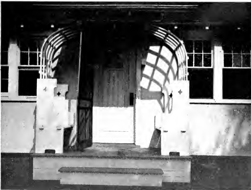
The entrance porch is not large, merely a small platform with seats sheltered by a vine lattice
