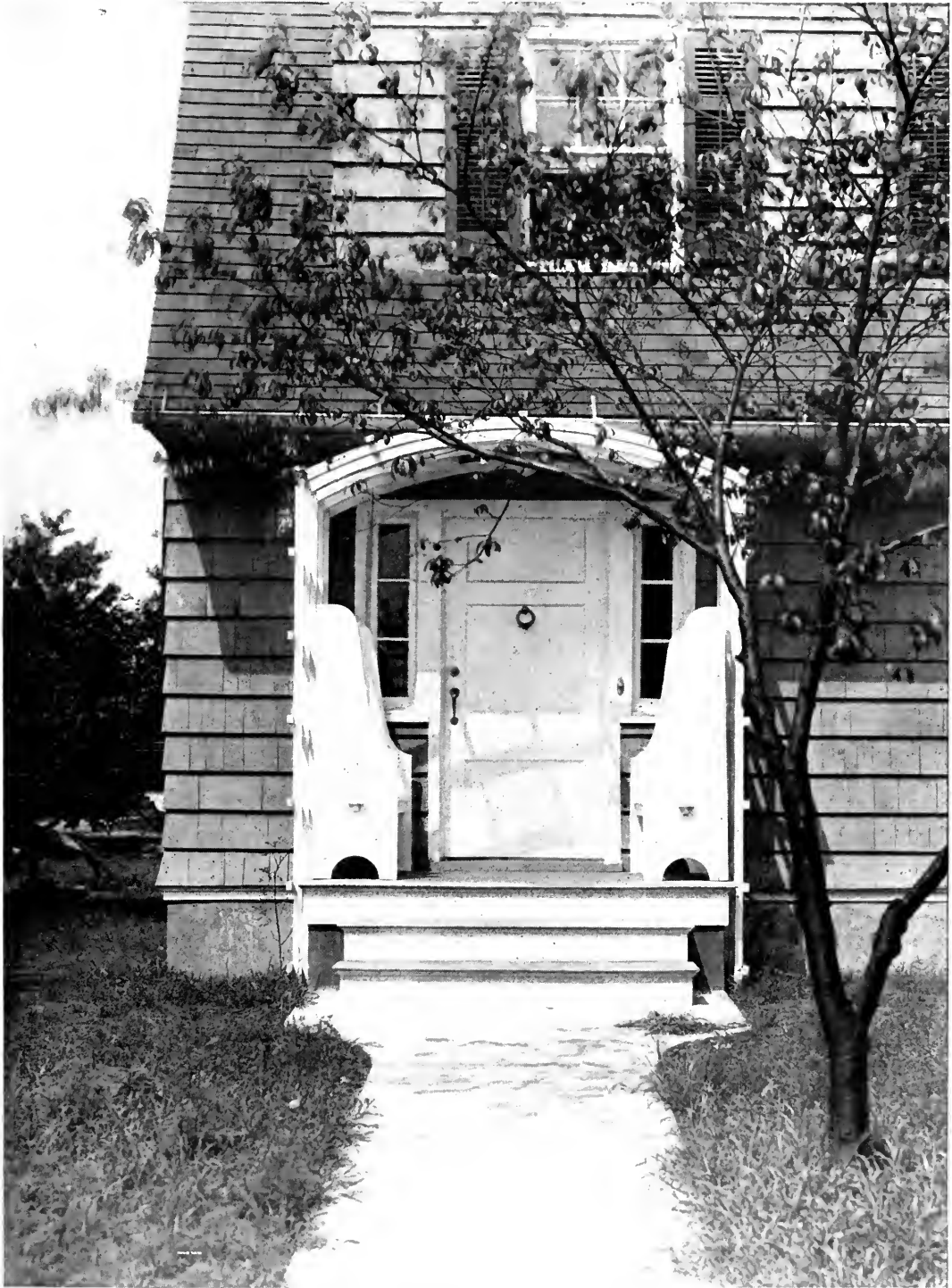
The house as built has widely spaced shingles stained silvery grey, with the outside woodwork white, excepting the second-story shutters which are green
