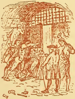
GATES IN BAD ORDER.
