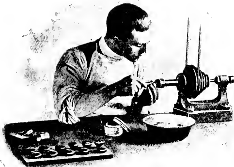
Fig. 535.—POLISHING LENSES.
