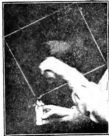
Fig. 145.—POURING OFF THE SURPLUS EMULSION.
