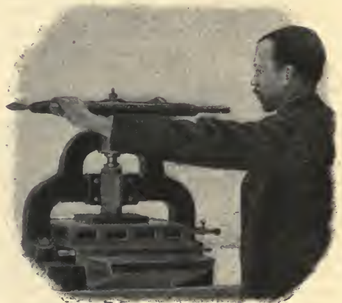
FIG 407.—MACHINE FOR DRY MOUNTING.
