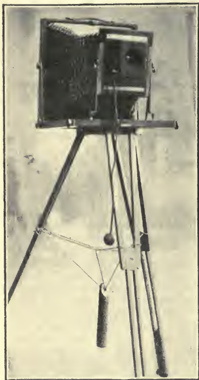
Fig. 790.—WEIGHTING THE STAND.
