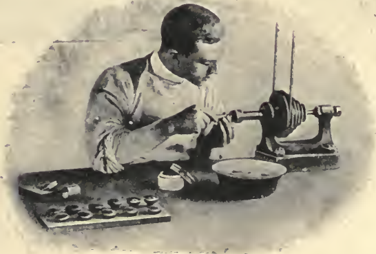
Fig. 535.—POLISHING LENSES.
