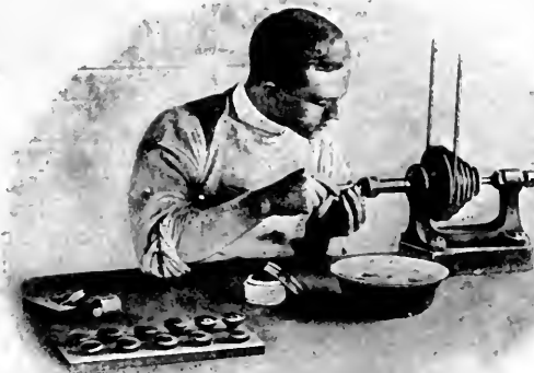
Fig. 535.—POLISHING LENSES.
