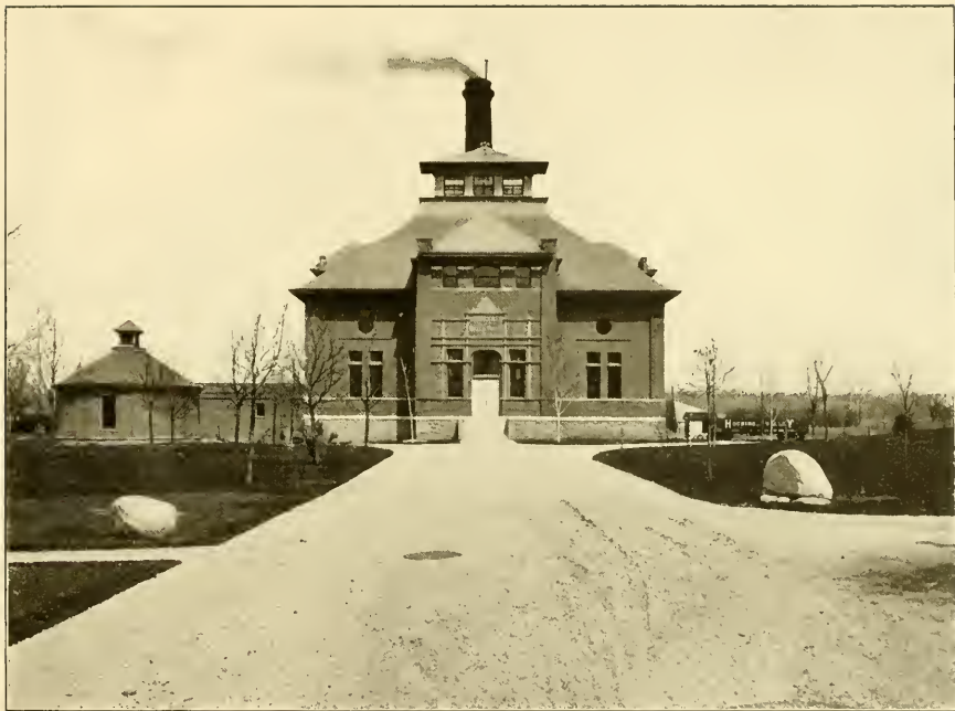
CITY WATER WORKS PUMPING STATION
