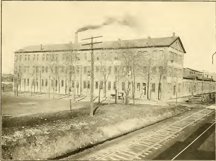
WIND MILLS, PUMP AND LAWN MOWER FACTORY
