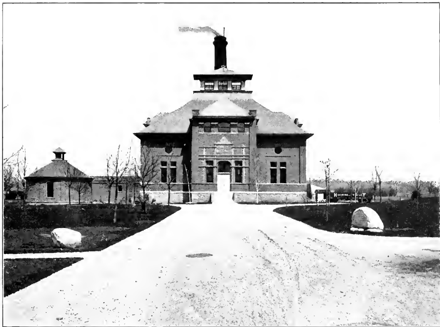
CITY WATER WORKS PUMPING STATION
