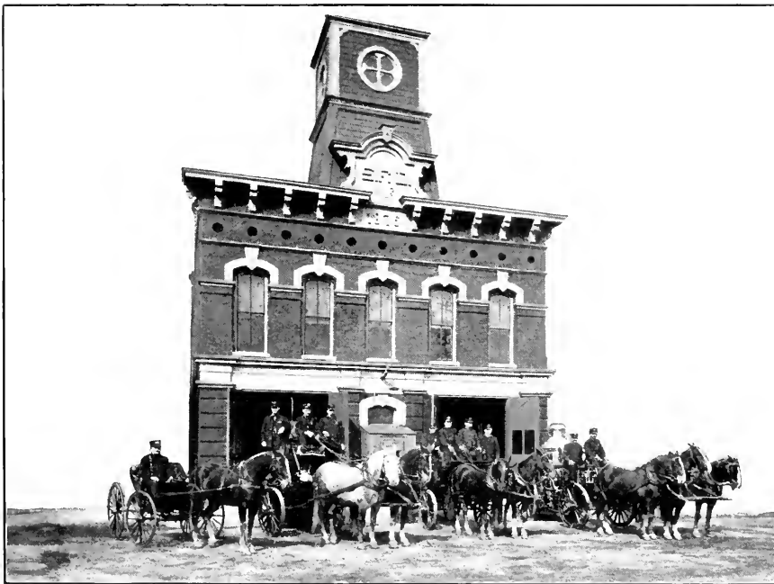
CENTRAL FIRE STATION
