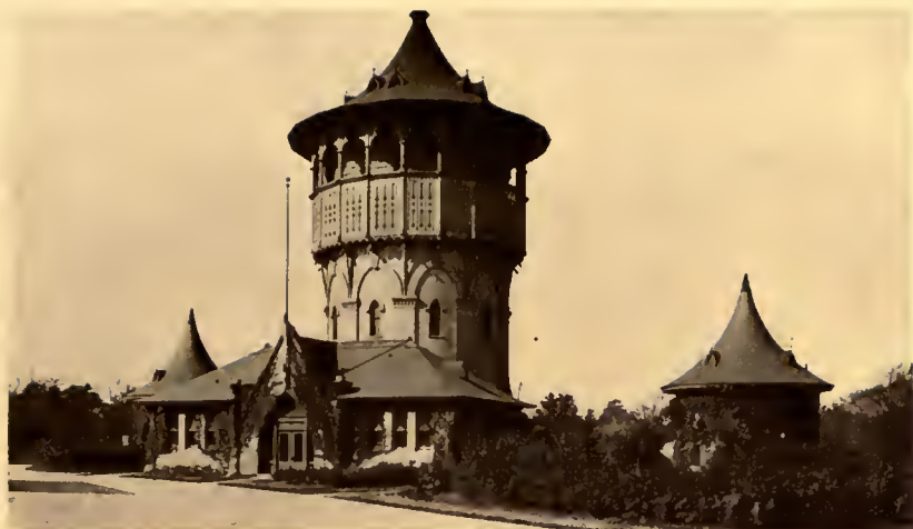
THE WATER WORKS Riverside, Ill.
