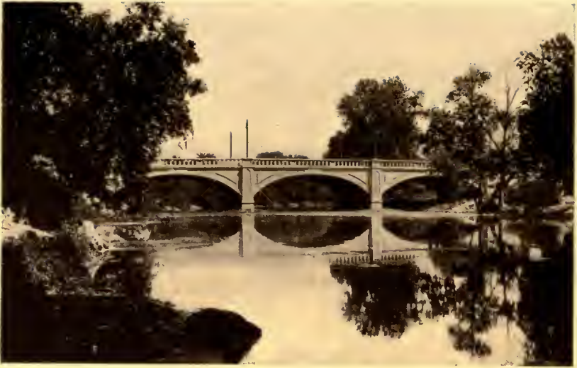
RIVER FOREST AND MAYWOOD New Bridge across the Desplaines on Lake St.
