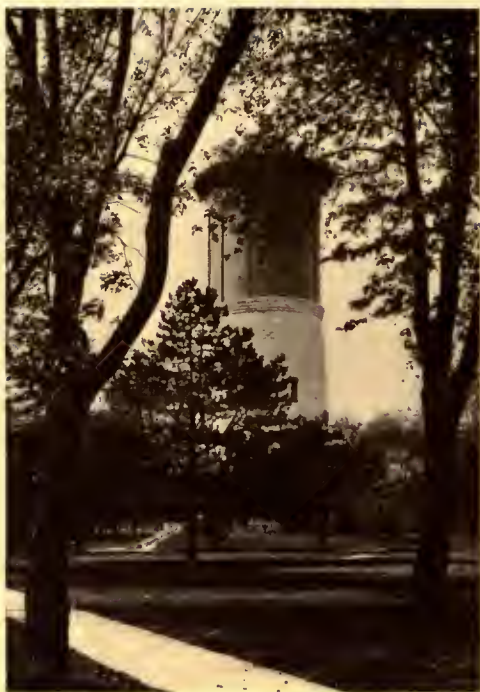
WATER TOWER Western Springs, Ill.
