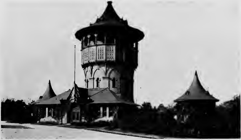
THE WATER WORKS Riverside, Ill.
