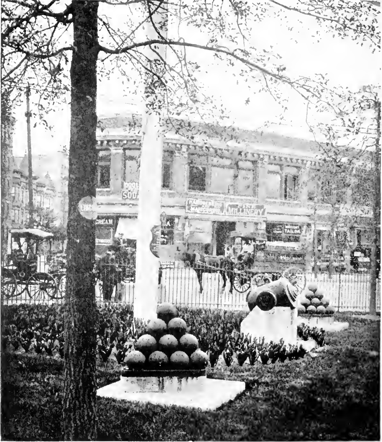
MCKINLEY SQUARE—169TH STREET AND BOSTON ROAD
