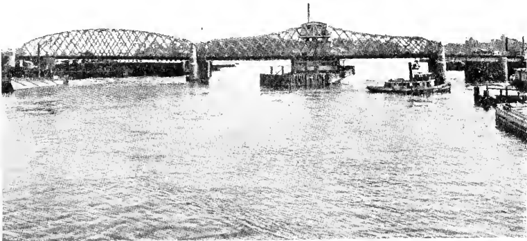
Courtesy Department of Bridges, City of New York
