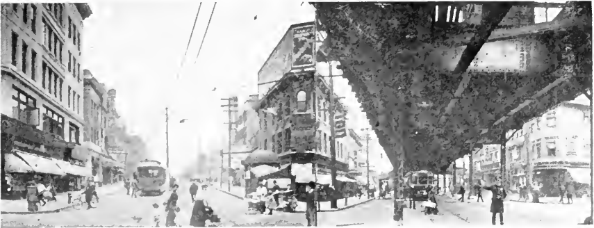
JUNCTION 149TH STREET AND THIRD AVENUE
