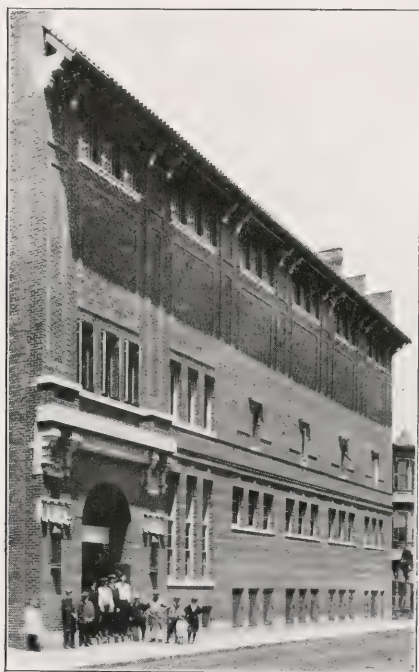
EAST BOSTON GYMNASIUM AND BATH.
