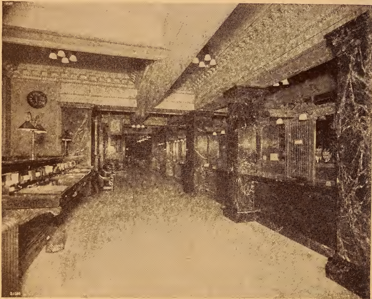
MAIN BANKING ROOM
