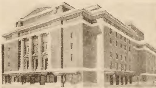
OPERA HOUSE—Plumbing by PIERCE & COX
