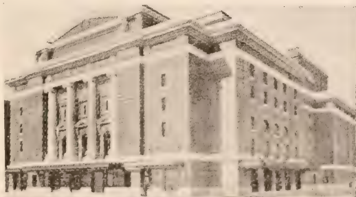
OPERA HOUSE—Plumbing by PIERCE & COX
