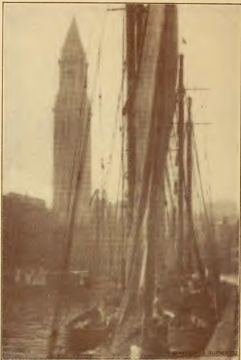
T WHARF AND CUSTOM HOUSE
