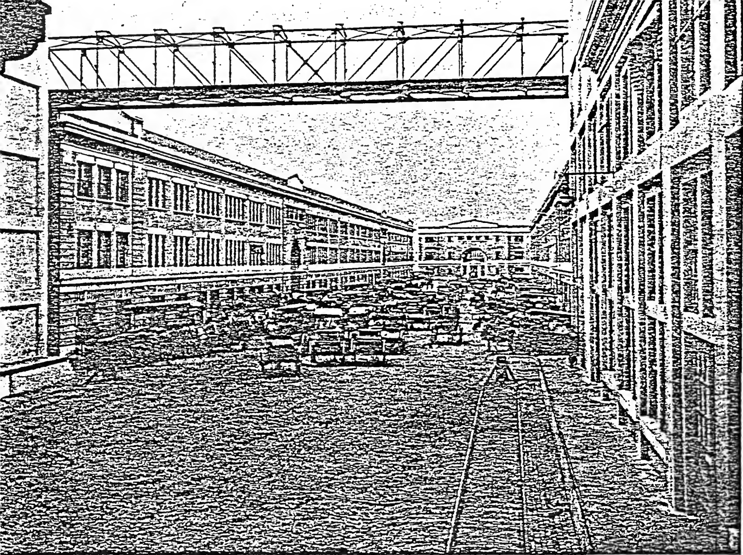
Boston Fish Pier
