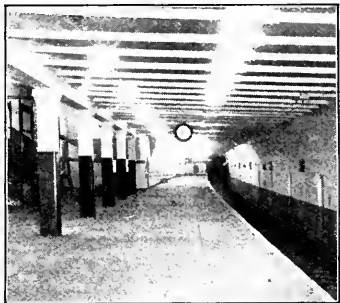
MILK STREET STATION, WASHINGTON STREET TUNNEL
