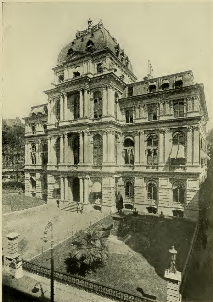
BOSTON CITY HALL, SCHOOL STREET.
