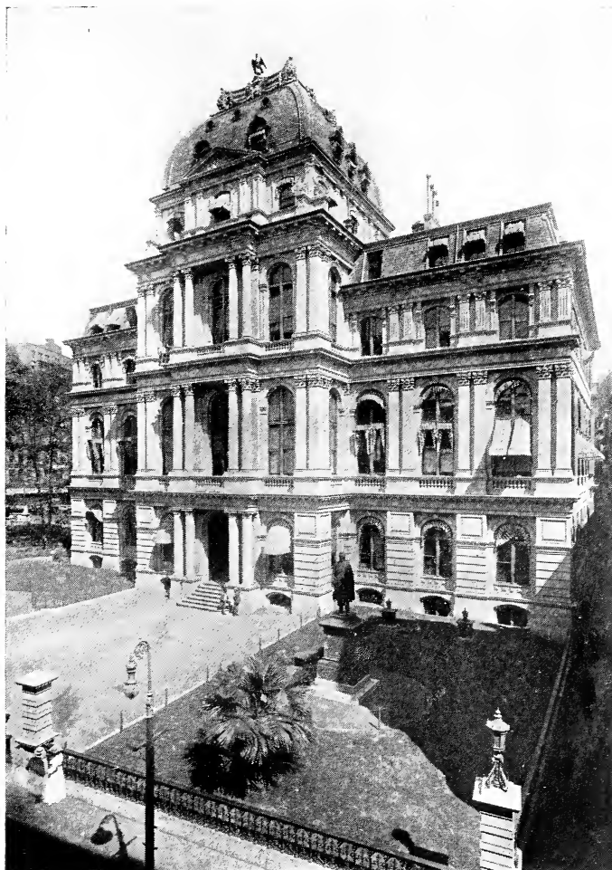
BOSTON CITY HALL, SCHOOL STREET.
