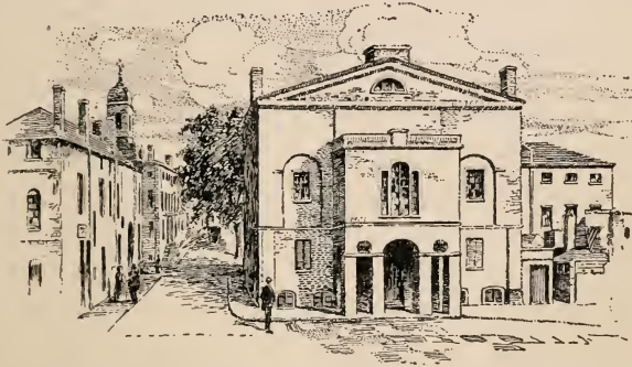
THE FEDERAL STREET THEATRE, CORNER OF FEDERAL AND FRANKLIN STREETS.
