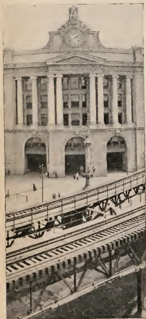
ENTRANCE TO SOUTH TERMINAL STATION.
