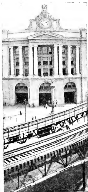
ENTRANCE TO SOUTH TERMINAL STATION.
