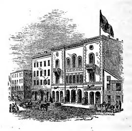
tablature and a pediment eighteen feet high at each end. The roof is covered with slate and zinc, and is surmounted by an octagonal lantern, twelve feet in diameter and eighteen feet high, having a window on each of its sides. The structure is covered on the exterior walls with cement,
