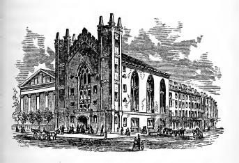
hammered granite, twelve feet high, with a belt of the same. The towers at the corners next Tremont Street are sixteen feet square, surmounted with granite battlements, and pinnacles rising ninety-five feet from the ground. The door and window frames are of fine ham-
