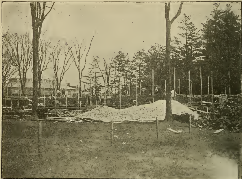
THE NEW DOMITORY IN PROCESS OF CONSTRUCTION
