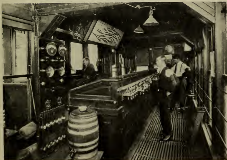
Inside the Terminal Tower where electricity does everything except the thinking
