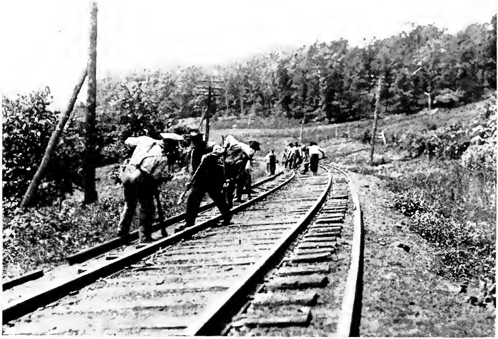
Changing rails between trains means hard work for the section gang
