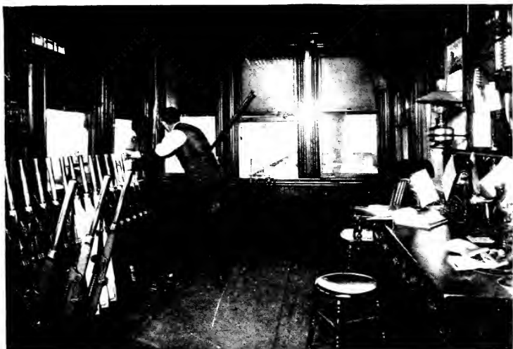
An old type of switch tower where switches and signals are turned by hand
