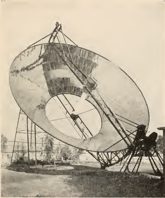
The Brilliant Steam Boiler Glistens in the Centre.
