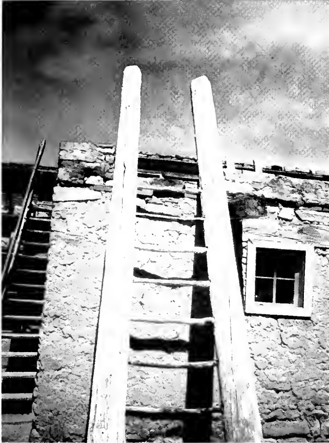
Above, ladder to a rooftop at Acoma
