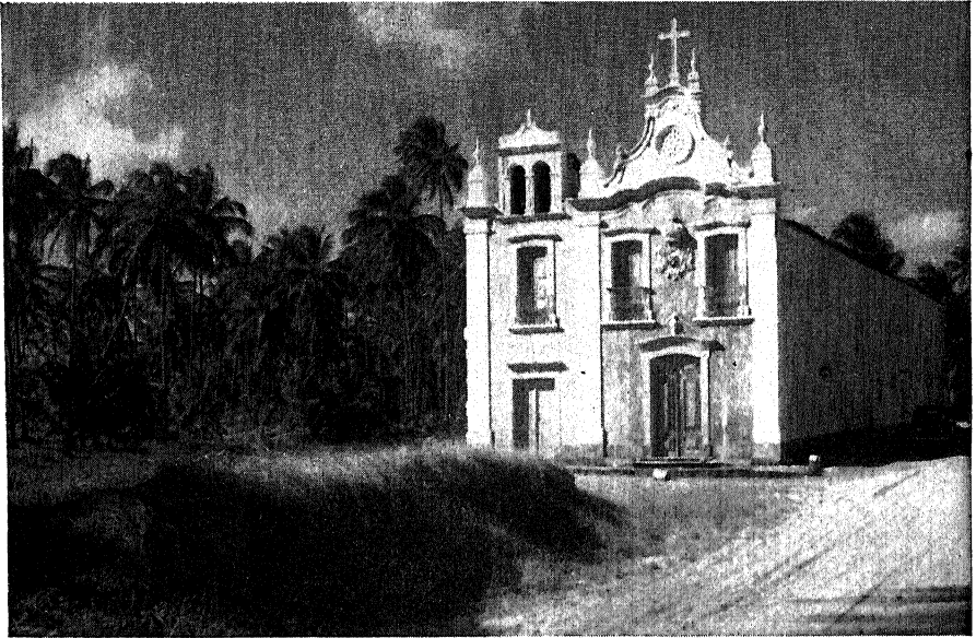
Early Portuguese settlers left their unmistakable mark on Brazilian buildings, as on this seventeenth century church in Recife, the principal city on the hump of Brazil and the site now of some of the hemisphere's most advanced business architecture.
