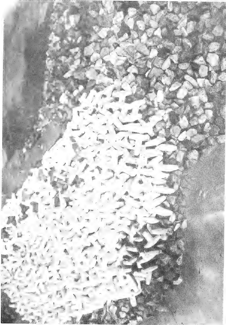
Photo 29. Special toe placement used for seaward transition of Plan 2B
