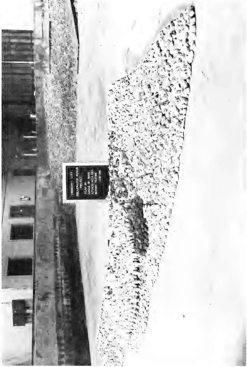
Photo 230. Seaward oblique view of Plan 26 before wave attack; 67.5-deg angle of wave attack
