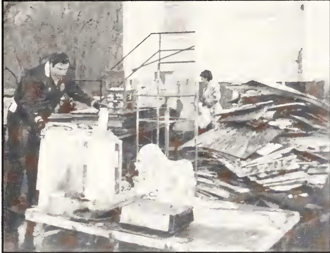
Cleaning out the basement.
