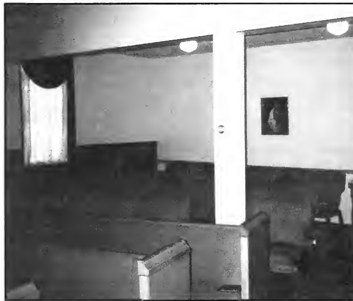
A view at the back of the remodeled sanctuary, where the wall was removed, showing upholstered pews and new chairs.
