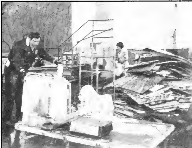
Cleaning out the basement.
