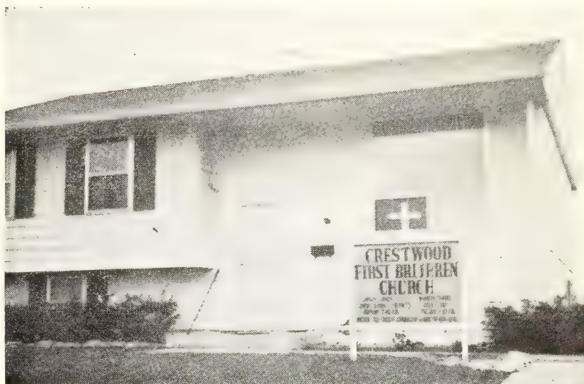
Crestwood Brethren Church in Fort Wayne, Indiana
