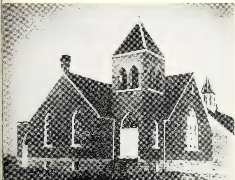
New Building replaces old (in background)
