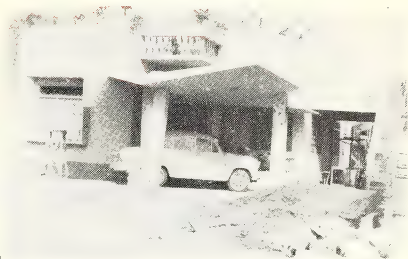
New home built by the Kumars in Rajahmundry
