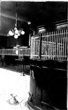
INTERIOR VIEW OF BANK.
