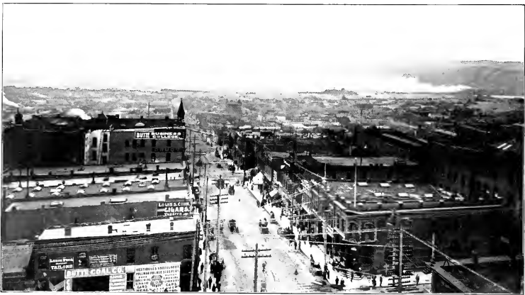
LOOKING SOUTH FROM CENTER OF CITY.
