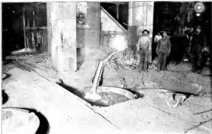
DRAWING OFF SLAG.
