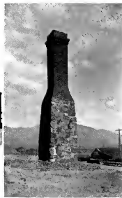
Stack of Centennial Smelter.
