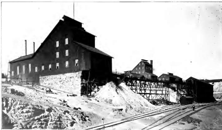
MOUNTAIN CONSOLIDATED NO. 2.
