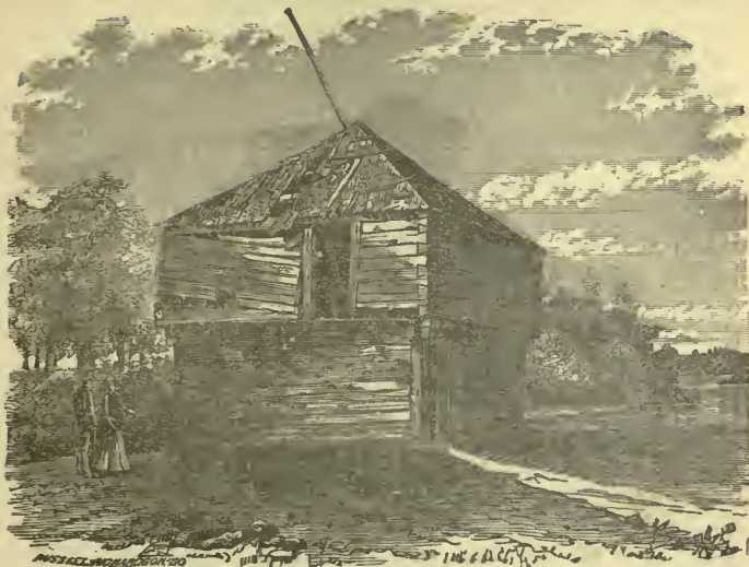
LAST BLOCK HOUSE OF FORT HALIFAX.
