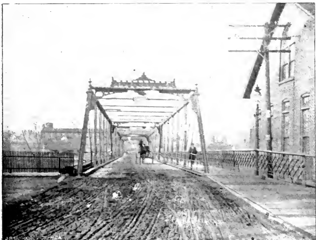
RIVER BRIDGE, EAST VIEW
