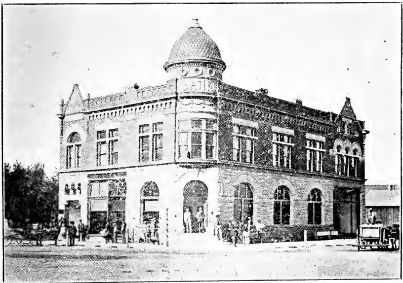
SPRINGVILLE BANKING COMPANY'S BUILDING, BUILT IN 1892.
