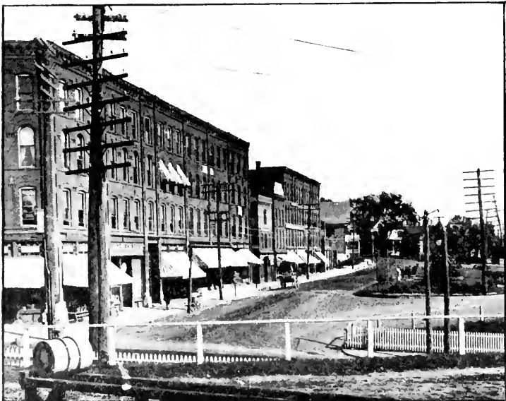
PROSPECT STREET, FROM R. R. BRIDGE.
