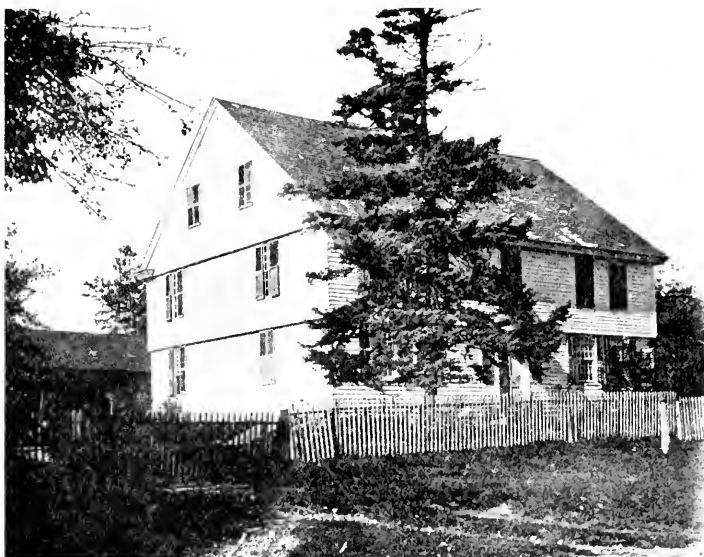
RESIDENCE BUILT BY WILLIAM (SECOND) AND BENJAMIN JEROME (NO. 37). SOLD TO ASA BARTHOLOMEW IN 1867, OWNED BY PHEBE (BRONSON) ALCOTT, OBERLIN O.
