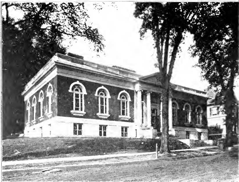
New Library Building.
