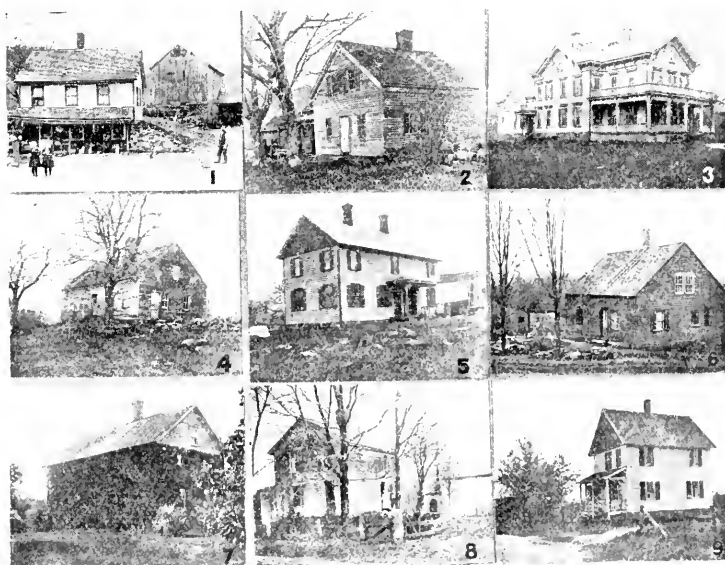
(1) No. 3, Mines Road, John Peterson O, The Michael Critchley Place ; (2) No. 2, Mines Road, L. S. Norton O, The Hiram Norton Place ; (3) No. 1, residence of L. S. Norton O, Site of the David Lewis and Joel Norton Places ; (4) No. 23, Stafford Ave., (unoccupied) The Theophilus Botsford Place ; (5) No. 21, Stevens St., Wm. H. Lugg O, The Philo Stevens Place ; (6) No. 22, Cor. Stafford Ave. and Stevens St., Mrs. R. W. Fox O, The Samuel Botsford Place ; (7) No. 24, Stevens St., Fred Carnell O, The Henry Smith Place ; (8) No. 40, Mix St., J. B. Sanford O, The John London Place ; (9) No. 39, Mix St., Mandus Carlson, The John London Place .
