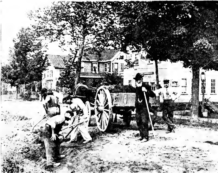
Street Department at Work.
