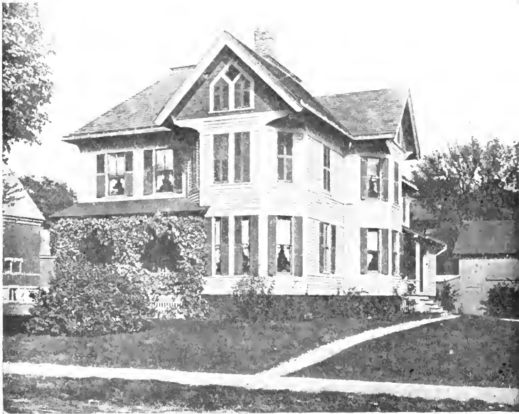
RESIDENCE REV. HENRY CLARK, CHURCH STREET.
