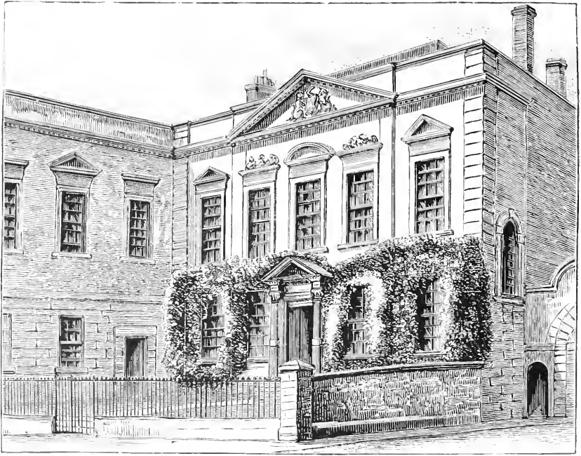
OLD CITY LIBRARY, KING STREET.
