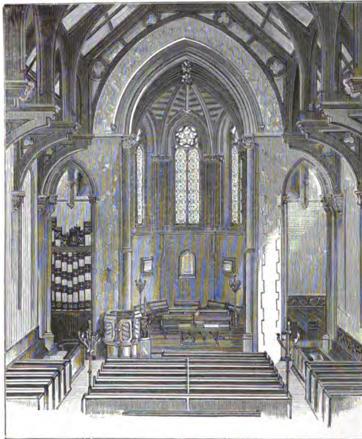
Interior of Clifton Down Congregational Church.
