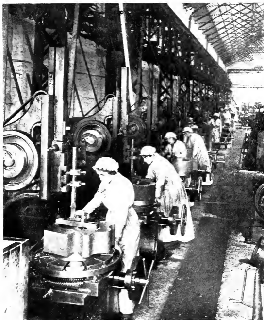
RANGE OF SLOTTING MACHINES ON 60-PDR. BREECH RINGS.
