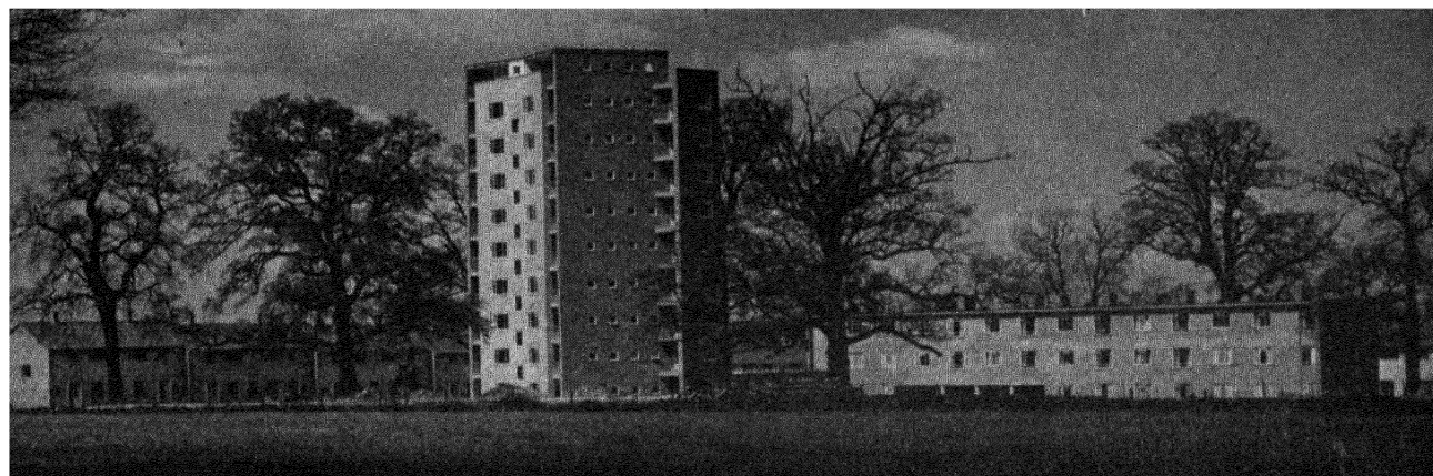
Blocks of flats, known as The Lawn , which were completed in 1951 at Harlow, Essex, one of the new towns being built around London. The flats would form part of the Mark Hall North neighbourhood of Harlow.
