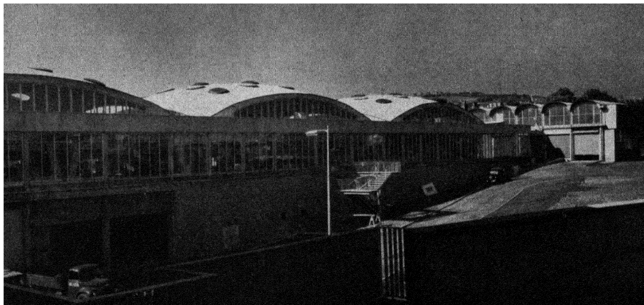
A large factory at Brynmawr, Breconshire, designed by the Architects Co-operative Partnership, which was completed in 1951.
