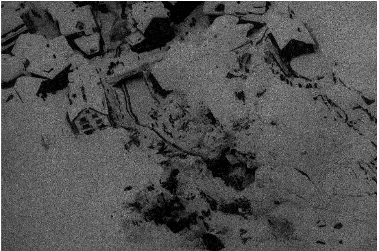
Early in 1951 many parts of Switzerland were severely damaged by avalanches. In Andermatt houses were buried and some of them were completely destroyed.
