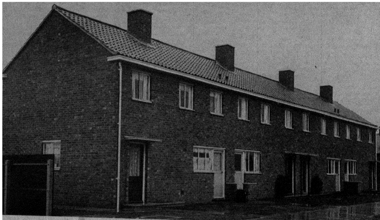
Houses built at Delapré, Northampton, in 1951 at a cost of £1,083 for each house. In Nov. 1951 "The Builder" (London) organized a competition for houses under £1,000 which was won by the borough architect and the deputy borough architect of the county borough of Northampton. The entrance and service doors are both at the front of the house.
