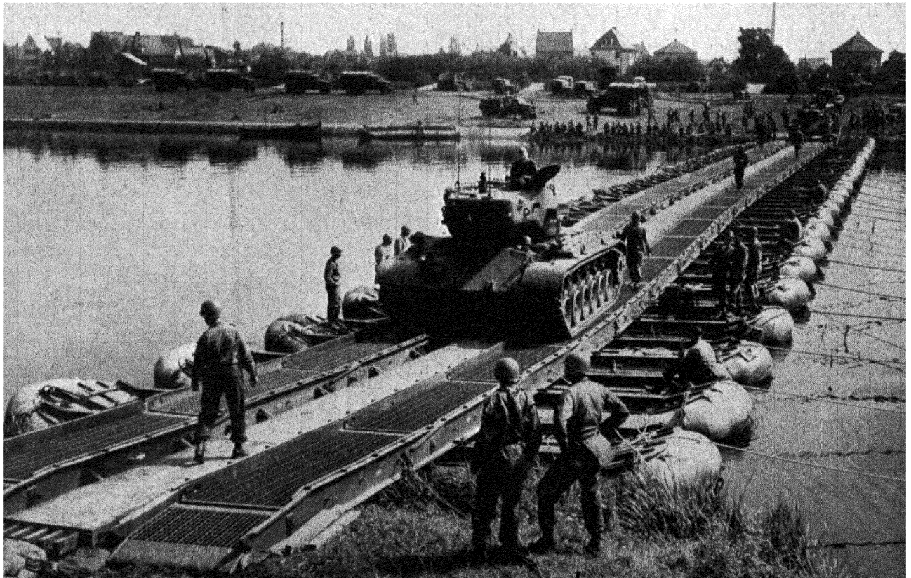
A pontoon bridge which was built in four hours across the River Main near Hanau, Germany, by troops of the U.S. 4th Division. The division arrived in Europe in 1951 to serve under General Dwight D. Eisenhower.
