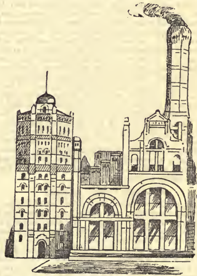
CORLISS ENGINEHOUSE AND WATER TOWER.
