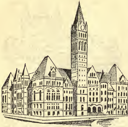
TORONTO MUNICIPAL BUILDINGS.
