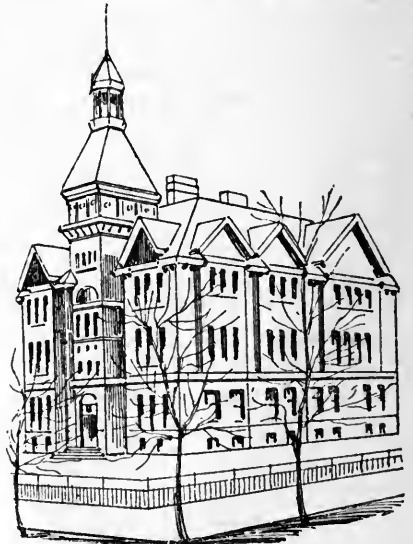
CHURCH STREET SCHOOL, TORONTO.
