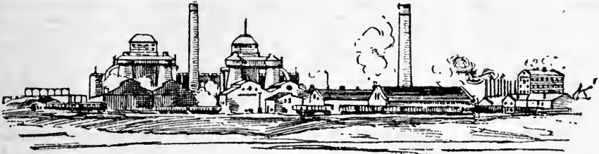
ILLINOIS STEEL COMPANY'S WORKS, NORTH PORTION.
